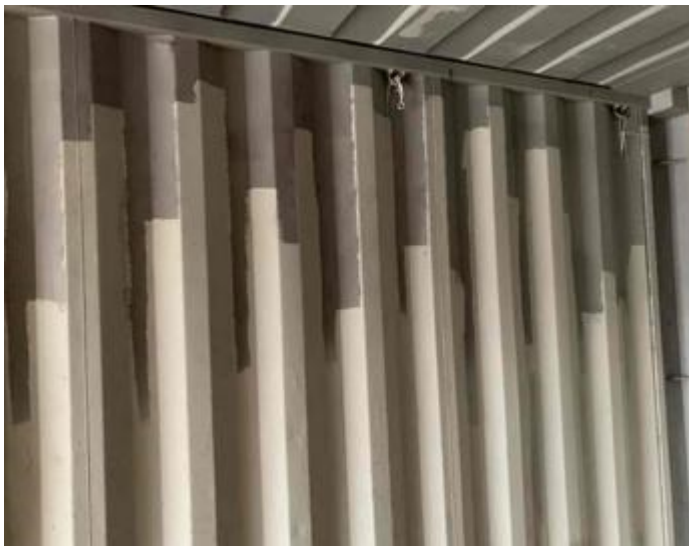
8.1.5. No defects inside container WALLS (Left & Right) 集装箱内侧面缺陷
