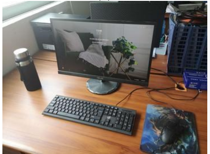
5.1. Telecom Equipment Available
