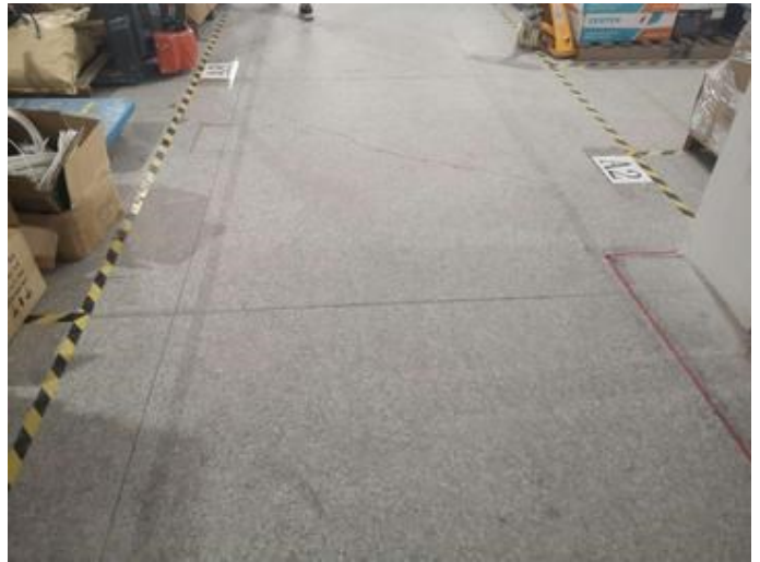
10.3. RM Warehouse Cleanliness
